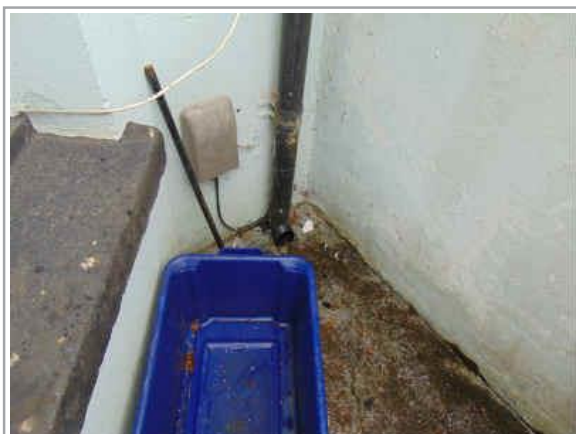
Rainwater pipe onto ground - front
