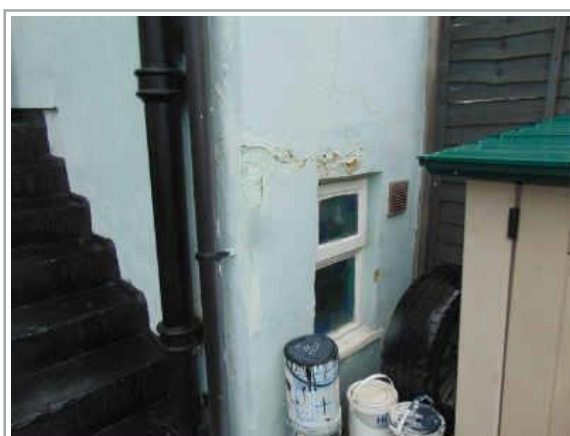
Defective render - decayed window
