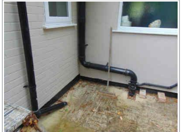
Soil and Vent Pipe
