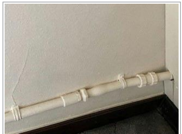
Lead/steel Pipework
