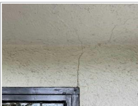
Cracking - Render
