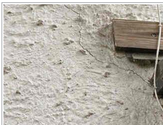
Cracking - Render
