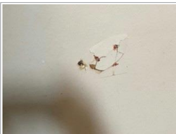
Localised Plaster Damage
