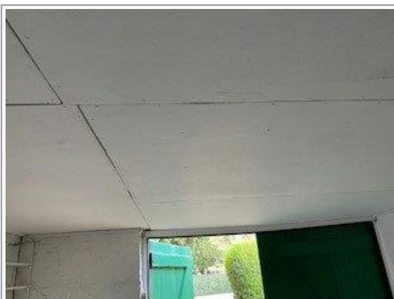
Ceiling - Possible Asbestos
