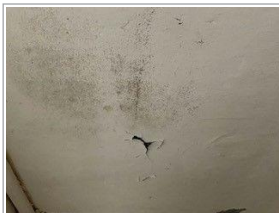
Condensation Staining
