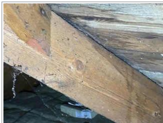
Staining - Roof Frame
