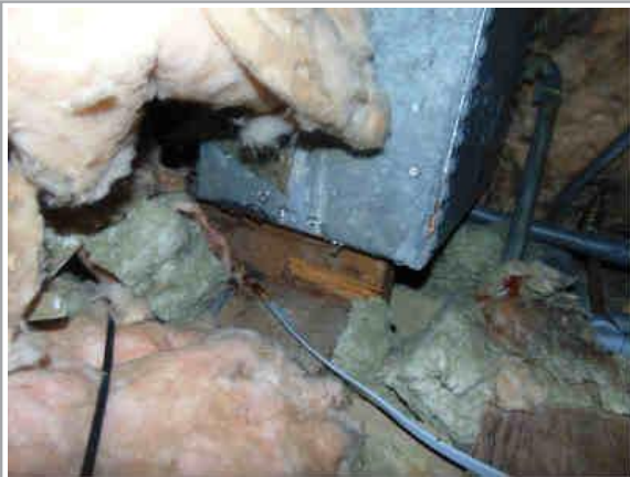
Corrosion - feed/expansion tank
