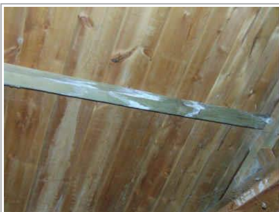
Old staining - roof timbers
