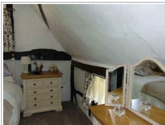
Crack - uneven ceiling
