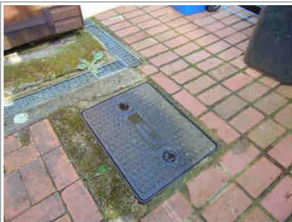
Drainage chamber
