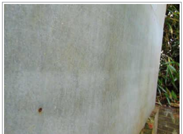
Fire protection - tank - possible asbestos
