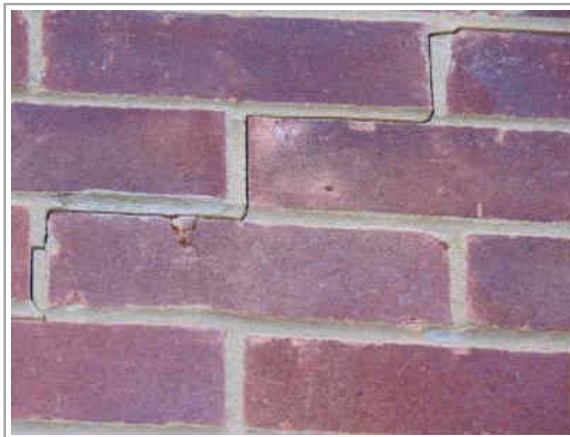
Cracking - rear elevation
