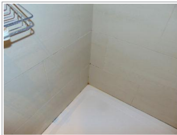
Mould on grout - shower room
